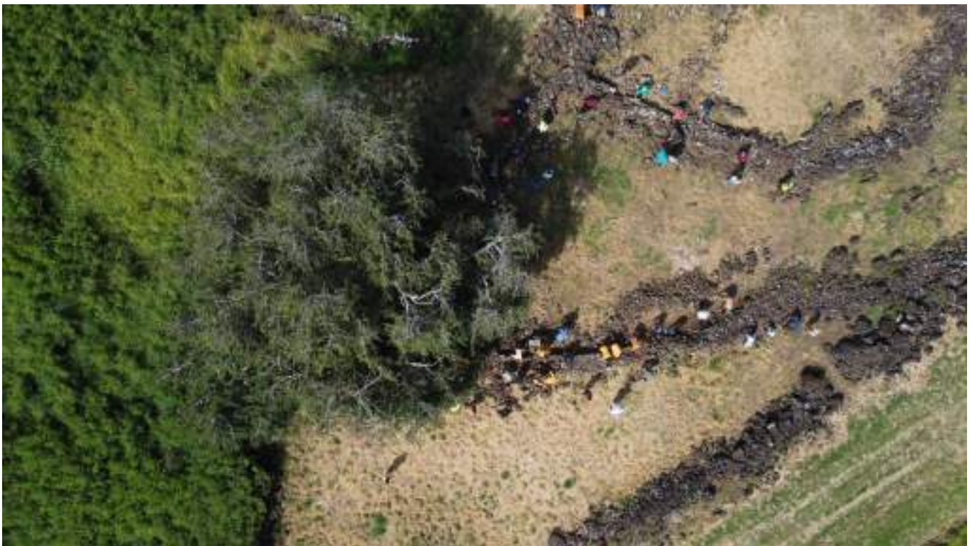
Fortifying the wall foundation at Hô'ai, Kaua'i at the Hui Malama Loko l'a Gathering 2023
